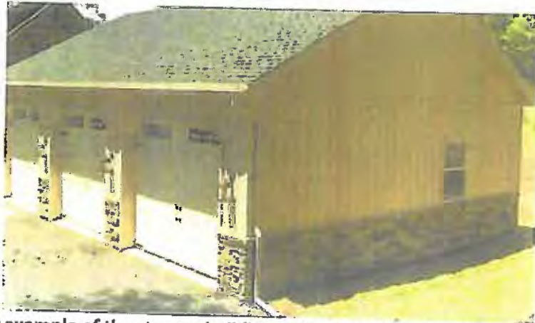
A similar example of the storage building style of stacked stone and metal siding.
