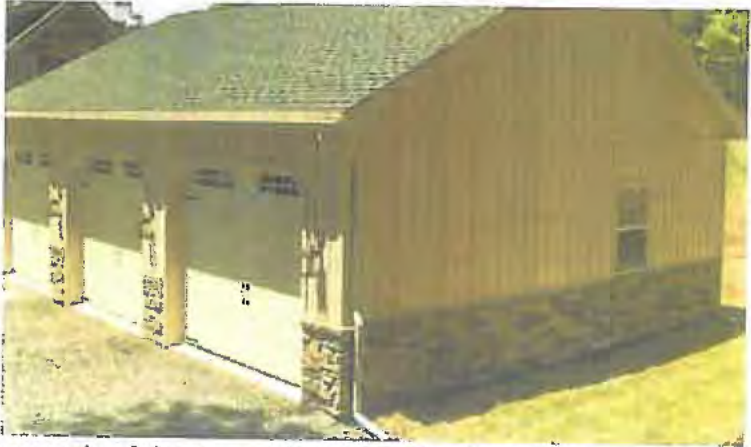
A similar example of the storage building style of stacked stone and metal siding.
