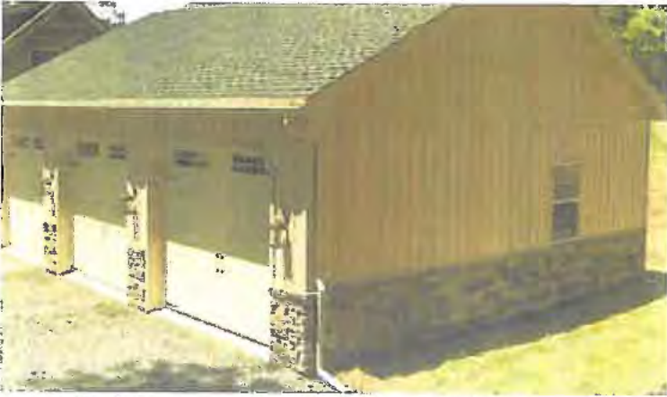
A similar example of the storage building style of stacked stone and metal siding.
